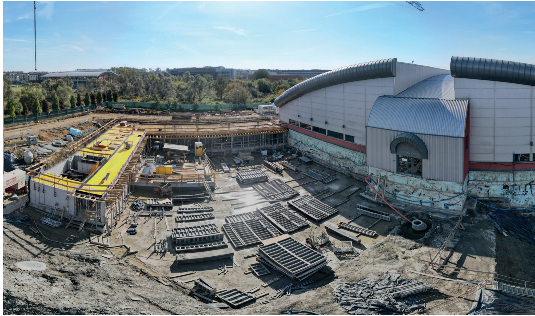
Photo 2. SOLARIS hall construction site. Photo: K. Adamczyk.
